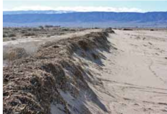
Figure 12: Berms are semi-permanent features on the landscape that provide effective reduction of blowing sand.
